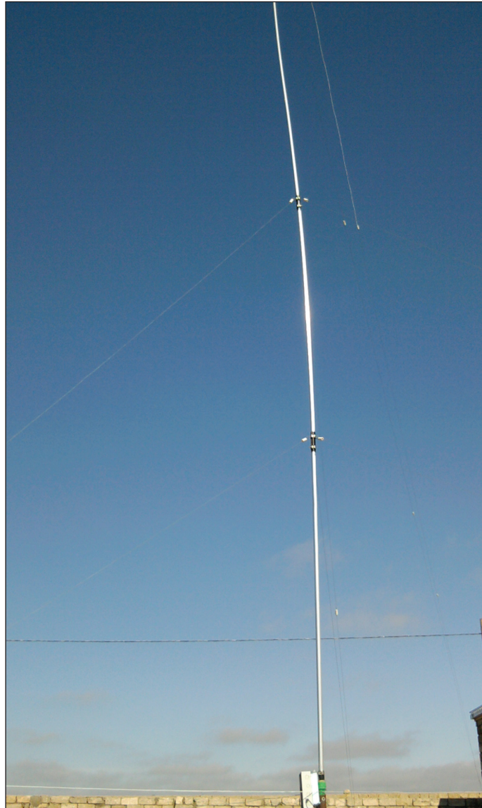
Antenna at 4K6FO
